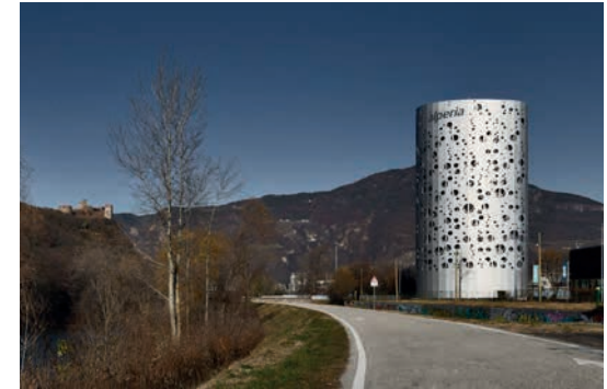
The new thermal storage tank at the Bolzano district heating plant, 40 meters high, with its plays of light architecturally enhances the entrance into the capital at night.
