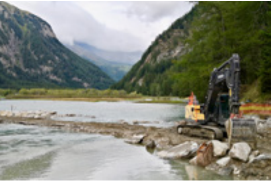
Removal of sediment in the Vizze basin
